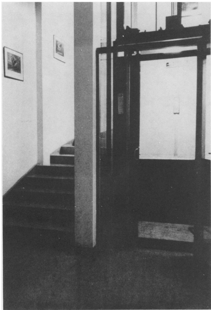
FIG. 6. —Elevator in Stonborough House, 1926–28. Note the exposed workings. From Bernhard Leitner, The Architecture of Ludwig Wittgenstein: A Documentation, with Excerpts from the Family Recollections by Hermine Wittgenstein , ed. Dennis Young (New York, 1976).
